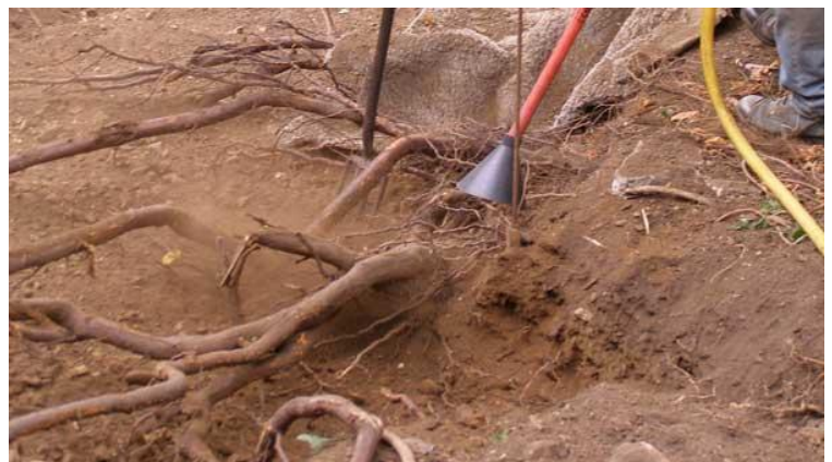
Air-Spade Exposes Roots for Transplanting
